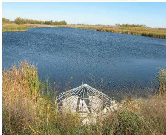
Odney Flaar Dam located in Onstad Township, Polk County
